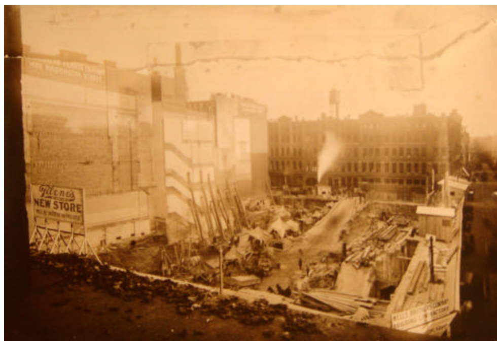
Corner of Washington and Summer streets following demolition of existing buildings, 1911. (source: Filene's Archives, Boston Public Library).
